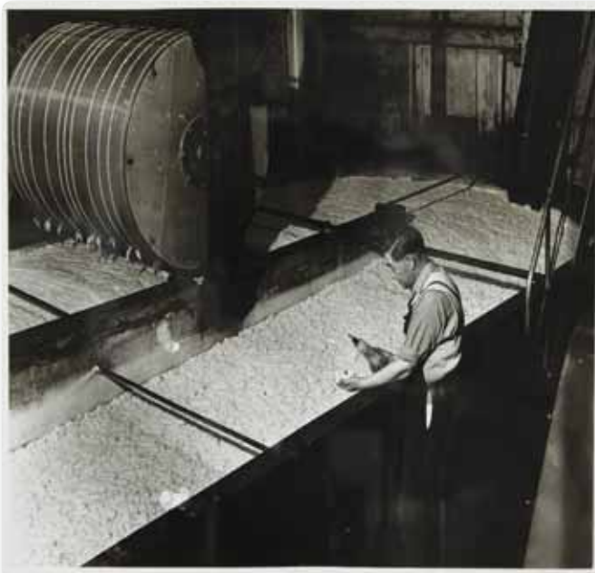
Attendant testing esparto pulp as it is being bleached (c1962) Reference ms38973/P/1. Courtesy of St Andrews University Library
