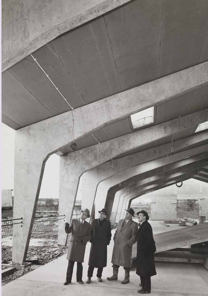
Inspection of building project using Crestone precast concrete, [1950s]. TCD MS 11482/4/2/18/12 © The Board of Trinity College Dublin
