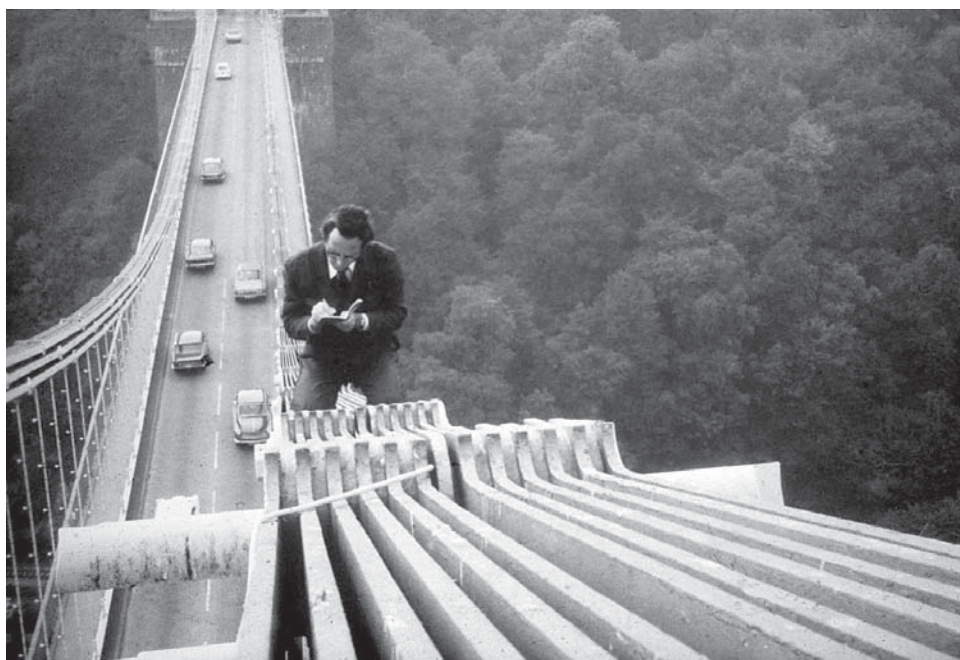
An engineer inspecting the bridge chains in 1973. Courtesy of CSBT
